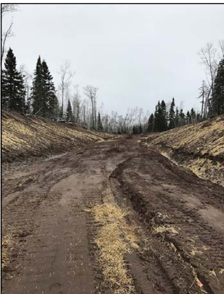
Rebuilt trail section at Temperance River Sate Park - April 2017 photo
